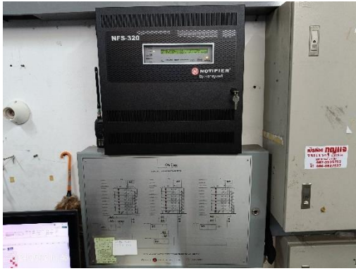
Fire Alarm Control Panel : FCP
