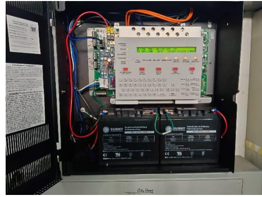
Fire Alarm Control Panel : FCP
